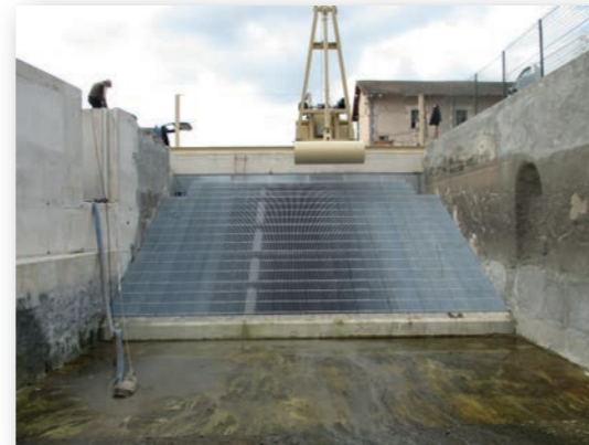
Racks 26° to the horizontal with downstream outflow
